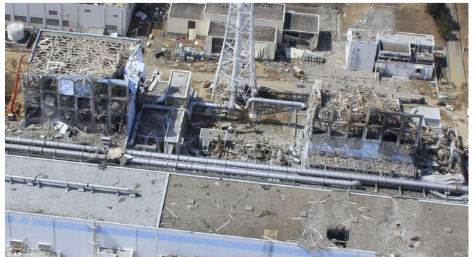
Fig. 3 An aerial view taken on March 24, Units 4 and 3 of the plant [27].
