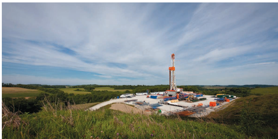
Drilling multiple horizontal wells from a single well pad allows access to as much as 1 square mile of shale that is located more than a mile below. [Image courtesy of Range Resources Appalachia]
