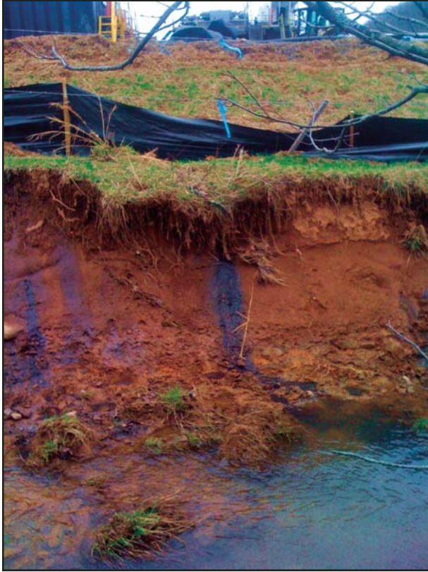
Figure 35. A black substance identified as drilling mud oozing out of the ground from an eroded stream bank below a drill pad and into the water of Indian Run in Harrison County, West Virginia, in 2010. Photograph is by Doug Mazer, used with permission.
