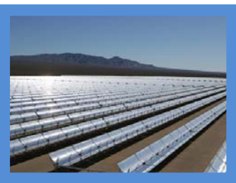
Nevada Solar One
