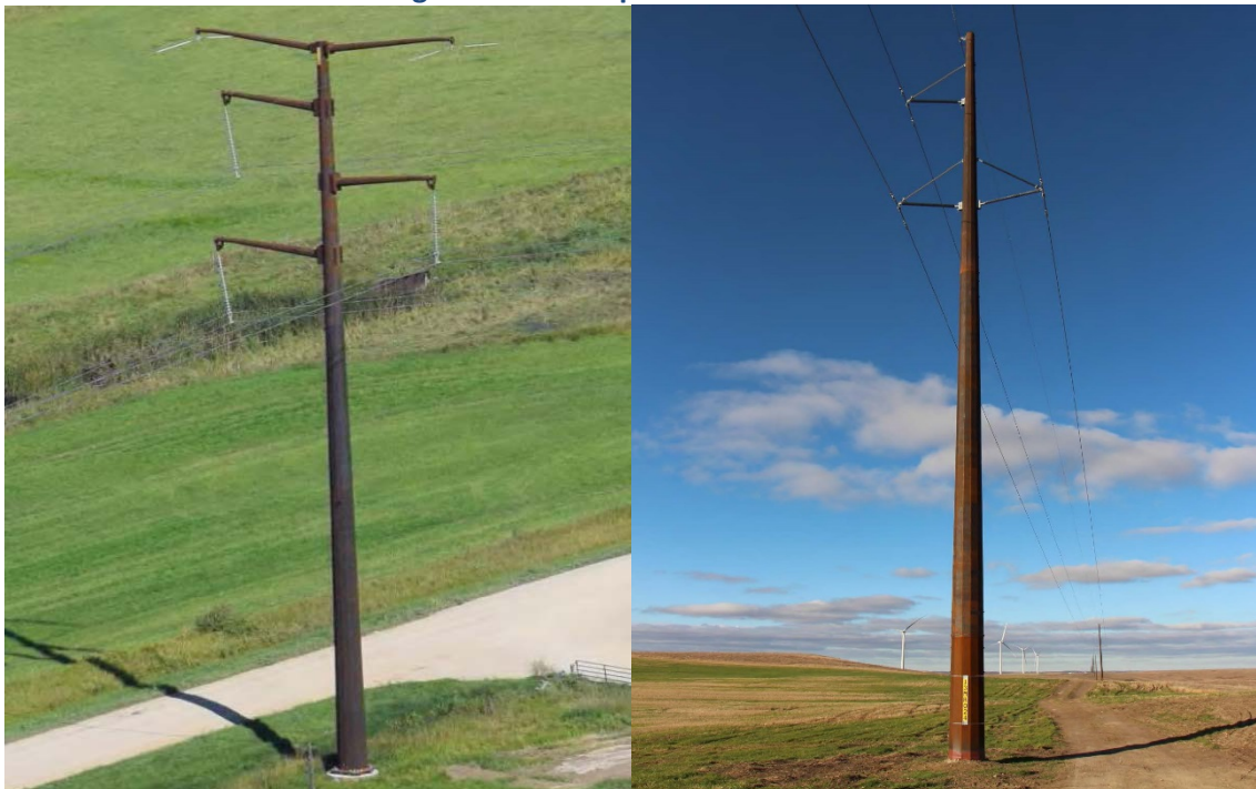
Diagram 13. Example of 345 kV Structures
