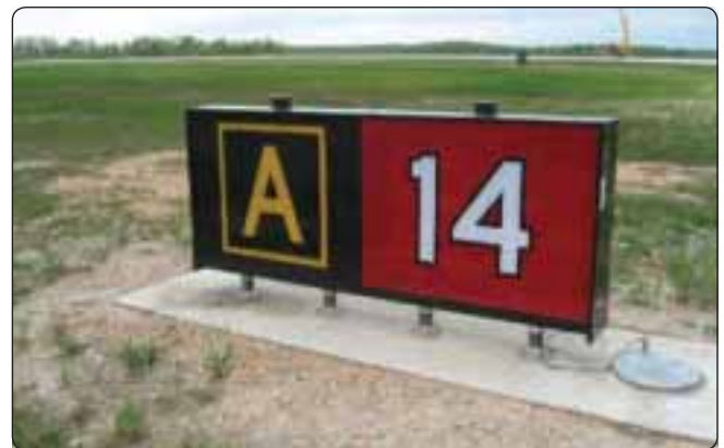
Figure 14-9. Runway holding position sign at takeoff end of Runway 14 with collocated Taxiway Alpha location sign.
