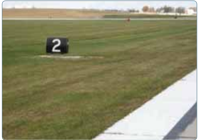
Figure 14-15. Runway distance remaining sign indicating that there is 2,000 feet of runway remaining.
