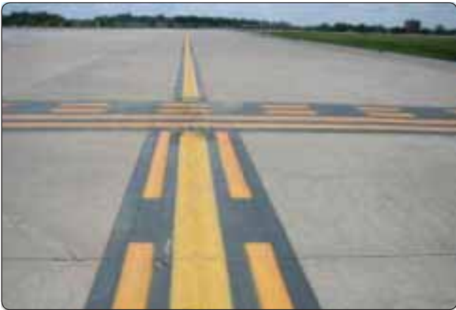
Figure 14-13. Surface painted holding position marking along with enhanced taxiway centerline.
